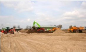
22 . Sitework progress is slow Fred Leopard Active , Normal 03. Construction phase , Terrain
